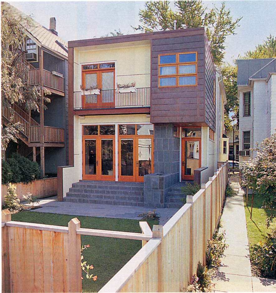
>> Cement board siding, copper shingles, and blue stone (above) give the back a geometric order. Responding to the owners' fondness for New Orleans, architect Richard Blender incorporated a balcony off the master bedroom and French doors leading to the garden. The palette complements the blue and creamy yellow of the front of the house (above right).
